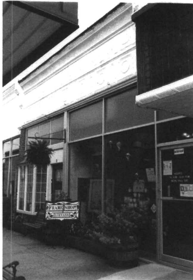
Figure Fourteen. The W. N. Evans Building, 1 Evans Arcade Photo by Becky Snider
