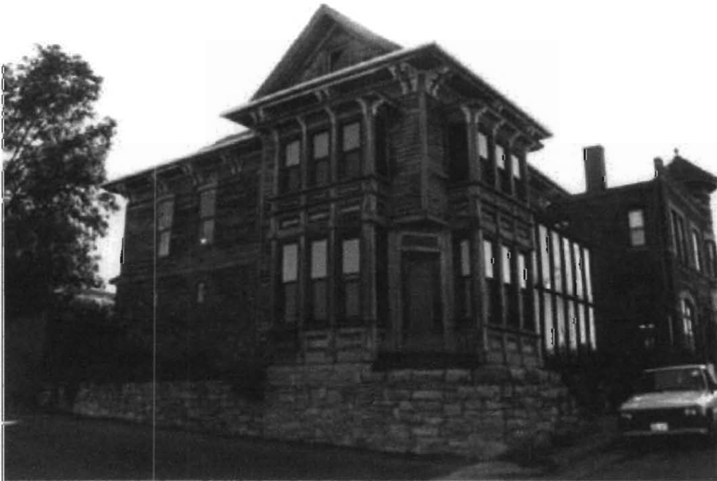
Figure Seven. The Joseph L. Thomas House in its current location at 104 Leyda St. Photo by Becky Snider
