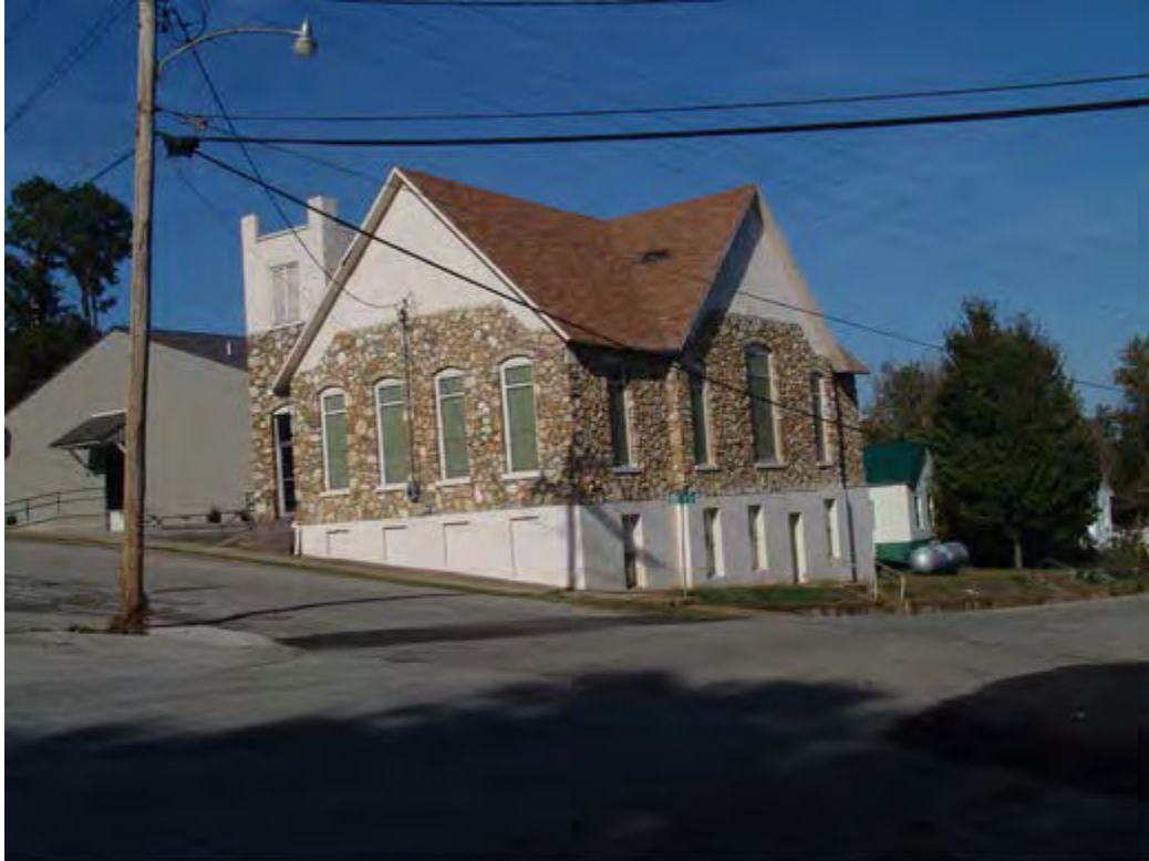
Figure 9: United Pentecostal Church 36.525279, -91.540895; Located at North 3 rd & Market Streets, in Thayer. Constructed c. 1920 by Otto & Frank Eder 39 . (Photo Source Kenneth Franke Oct. 2016).
