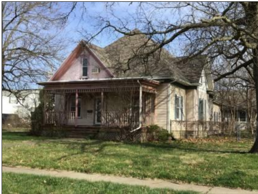
Figure 33. This high-style Queen Anne at 701 E. Harrison Street features an irregular shape and hip and gable roof. The porch features turned wood posts and spindlework.
