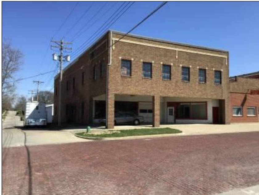
Figure 50. Chicago-style commercial building at 514 North Franklin Street.
