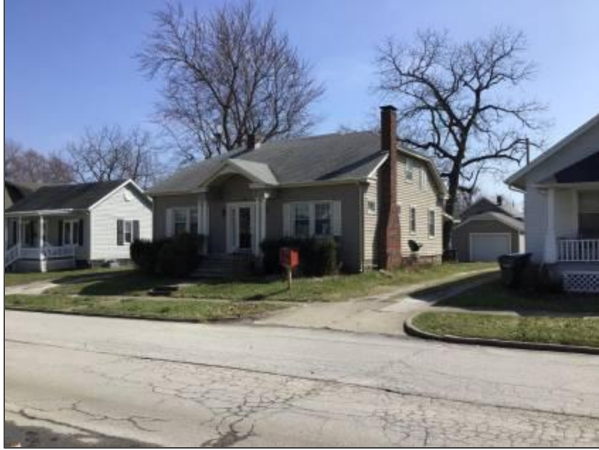
Figure 36. A later Colonial Revival example at 810 East McPherson Street.
