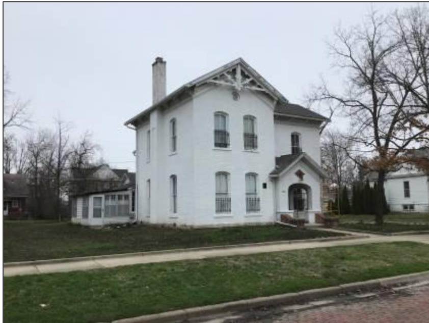
Figure 47. Italianate-style house at 415 East Washington Street.
