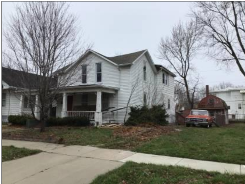
Figure 22. Center gable form house with Craftsman porch details.
