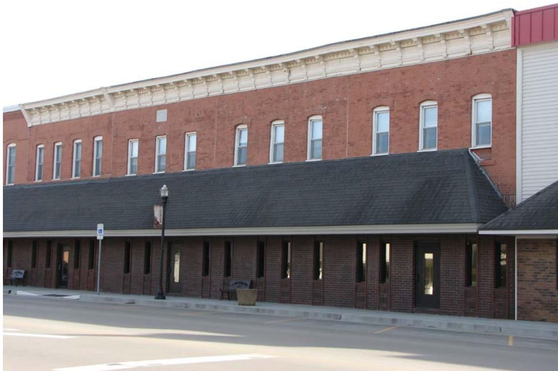
Figure 8. 110-116 W. 4th Street has been altered on the first-story level. The upper portion of this commercial row retains sufficient integrity to be considered contributing to the downtown commercial district. View is southeast (Photo: Ruth Keenoy, 16 February 2018).
