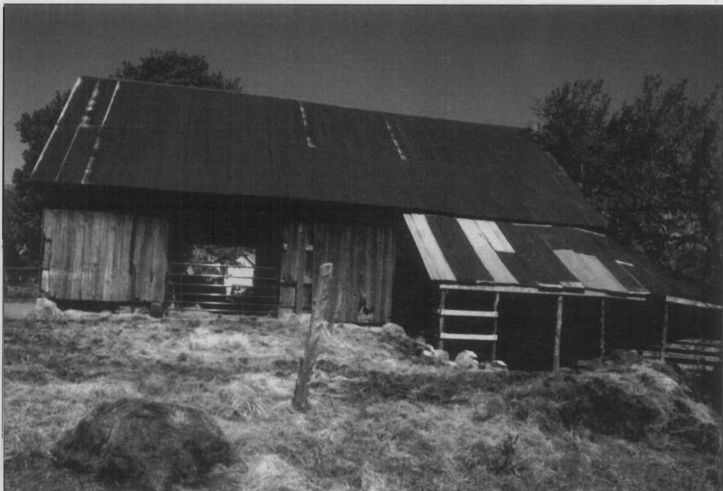
Cedarcroft's East Barn at the conclusion of the work.
