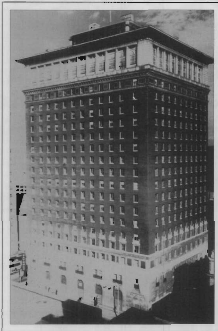
The Hotel Statler (1917) is listed in the National Register of Historic Places as a significant example of the innovative designs of George B. Post & Sons, the New York firm that set the standard for modern hotel design. Although currently vacant and threatened by possible sale for demolition and new construction, the Statler appears to be in good condition and remains highly intact.
