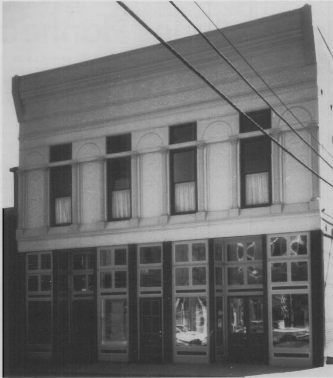
Historic Clarksville, Inc.'s most recent project was the former I.O.O.F. Hall. The second story meeting room now serves as a community center. A new elevator (only the second in the county) provides accessibility.
