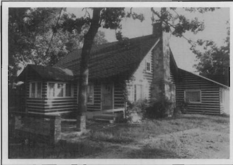
This former summer place in Forsyth is a good example of typical slab log cabin construction. Note the characteristic white Portland Cement chinking between the logs.
