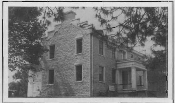
The Ste. Genevieve Academy, ca 1808-1810, may be the nation's oldest school building west of the Mississippi.
