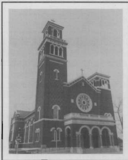
Built in 1922-23, Our Lady of Sorrows Catholic Church, Kansas City, was designed by Henry W. Brinkman of Emporia, Kansas. Brinkman specialized in church architecture and designed many religious structures in both Missouri and Kansas. Photo courtesy the Kansas City Landmarks Commission.
