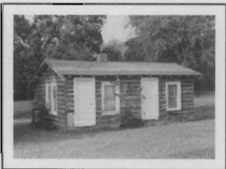
A half-log veneer gives the Hardesty cabin (ca 1930) its rustic appearance. Part of a three-building complex that also included a filling station and garage, the cabin was once rented to travelers passing through Avilla overnight on Route 66.
