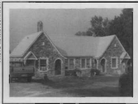
This four-unit building at the Wagon Wheel Motel is constructed of rubblestone in the English Cottage style. Note the window and door trim of white glazed brick. Located in Cuba, Crawford County.
