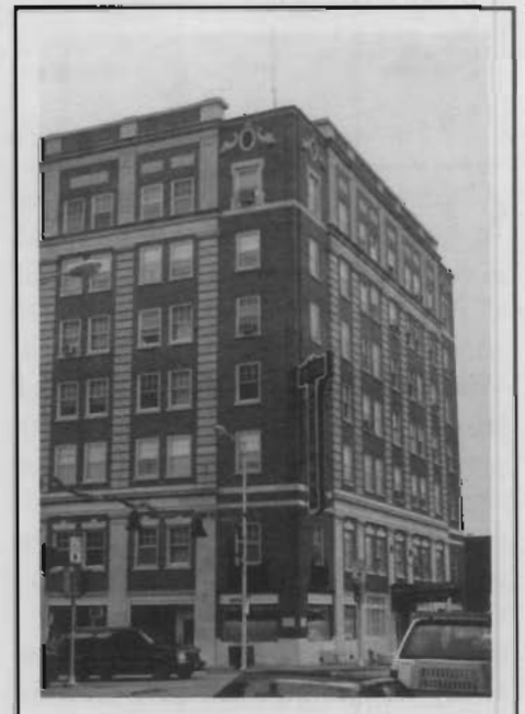
Historic Hotel Bothwell in Sedalia was successfully adapted for use as senior citizen apartments.
