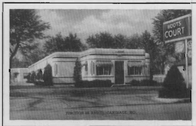
The Boots Motel, constructed in 1939 and shown on this historic postcard ca 1945, is a good example of the Streamline Moderne style. Note the rounded corners and roof parapet emphasized by bands of black tile by day and neon tubing by night. Located in Carthage, Jasper County. (Courtesy Route 66 Association, Jim Powell.)
