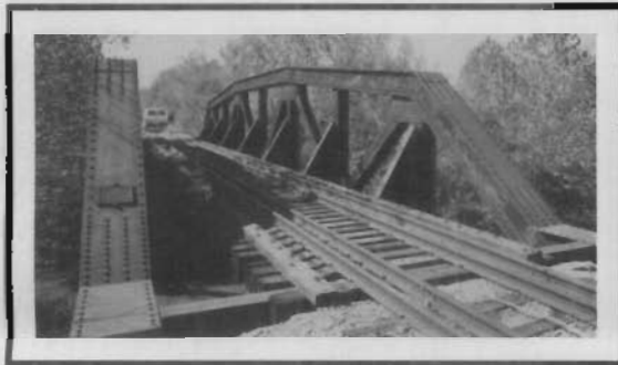
MKT Bridge #13 crosses Sand Creek in Henry County. It is a Warren with verticals, pony truss with an unusual polygonal top chord which has exactly five slopes as in a camelback. Notice even in this diminutive form the verticals carry the sway bracing. The bridge was built in 1926 by the American Bridge Company.
