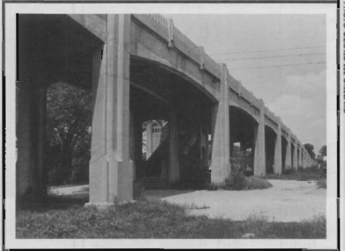
The Highway 5 Bridge over the Katy Trail is located near New Franklin in Howard County. This early 20th-century bridge illustrates a closed-spandrel, reinforced-concrete arched bridge.
