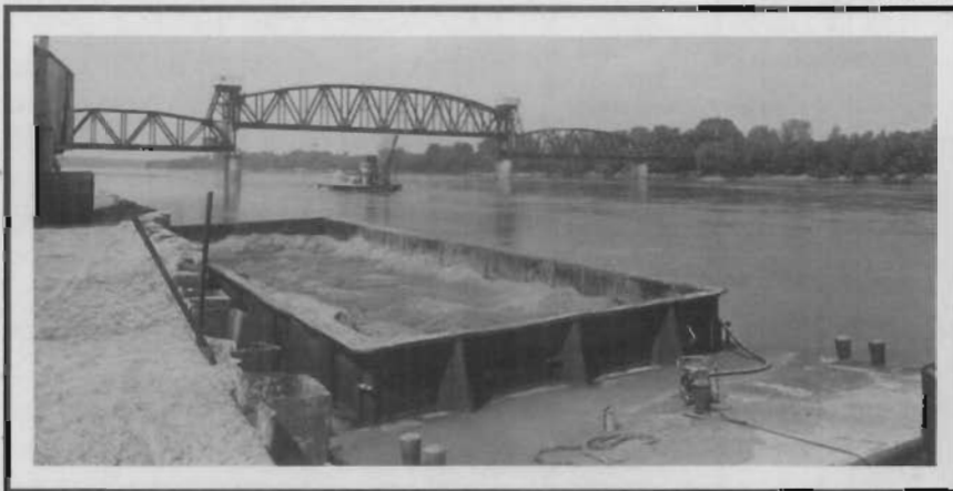
MKT Bridge #3 at Boonville spans the Missouri River linking Howard and Cooper counties. It was built by the American Bridge Company in 1930-31. Besides having four truss spans totaling 1,147 feet, which help make it the longest MKT bridge, it also has a 408-foot lift span which, when built, was the longest in the world.
