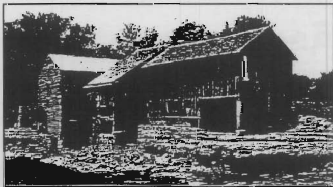
Although it was demolished in 1953, the stone foundations of the old Fitzhugh-Watts' Mill (1834) remain on the west bank of Indian Creek at 103rd Street in South Kansas City. The mill site is being nominated to the National Register for its association with the Santa Fe Trail. Photo courtesy of Jackson County's Historical Society Archives.
