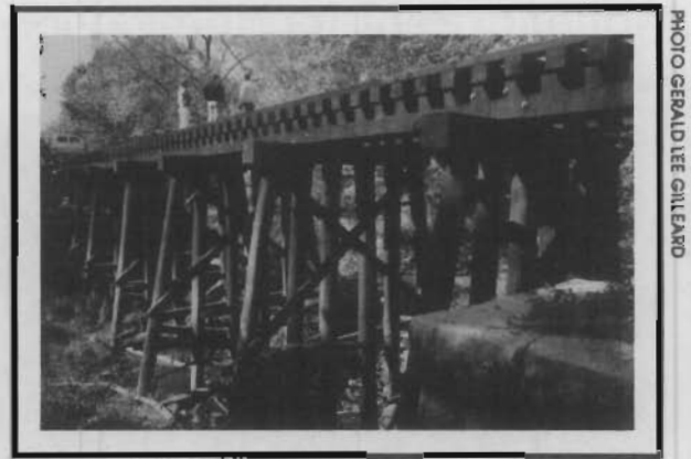
MKT Trestle (8) crossing a branch of Tebo Creek in Henry County is an open-deck, timber trestle. It appears to be of recent construction.
