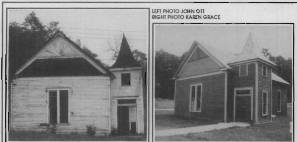
The Mount Nebo Baptist Church, Rocheport, Boone County, before and after its rehabilitation as an Investment Tax Credit project. Note the leaning bell tower in the before photo (left) and the dramatic change in the after photo (right).
