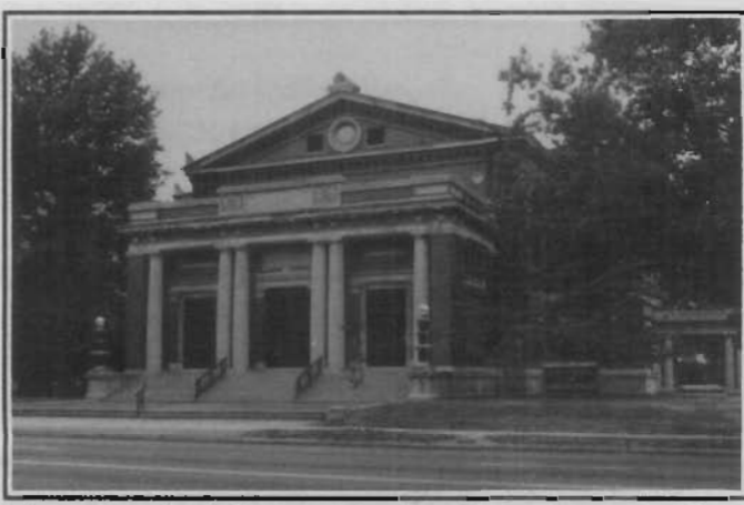
First Church of Christ, Scientist, St. Louis, designed by Mauran, Russell and Garden, 1903 is listed in the Holy Corners National Register Historic District.
