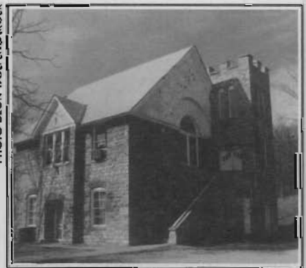
Completed in 1907, the Washington Chapel CME Church in Parkville interprets the late Gothic Revival style in locally quarried limestone.
