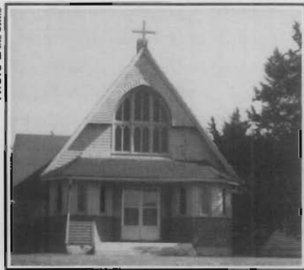
St. Oswald's Protestant Episcopal Church, ca 1892, located in rural Atchison County, is an example of the Shingle style of architecture.
