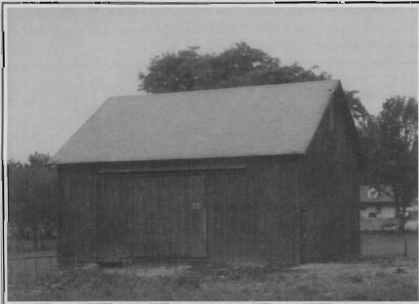
This English Barn was built prior to the Civil War on the farm of Greene M. Shelton. It sits on a stone basement and is held together with hickory pegs. Located in Grandview, Jackson County.
