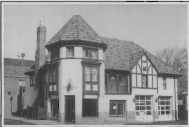
Designed by H.A. Pope & Sons, Inc. in 1931, this French Eclectic style station reflects the belief of the City Beautiful movement that station design be compatible with the surrounding neighborhood. Located in University City, St. Louis County.
