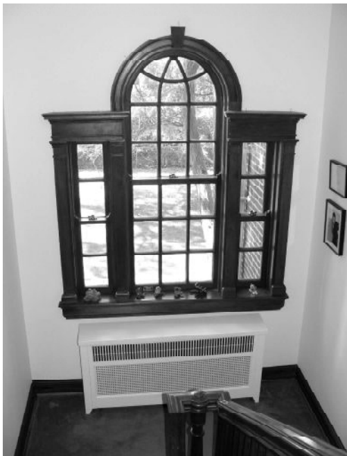
Image P Palladian window on staircase landing.
