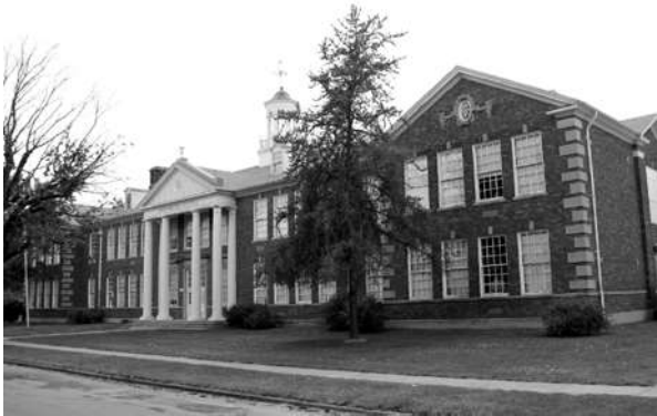
Figure EE Greenwood Elementary School (1934-1935).
