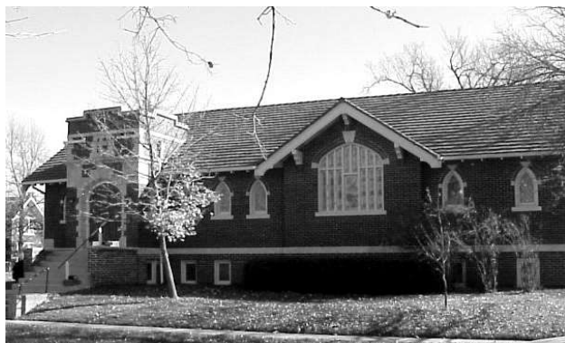
Figure V Trinity Episcopal Church (1917. NR Listed 01/02/08), Private photograph.
