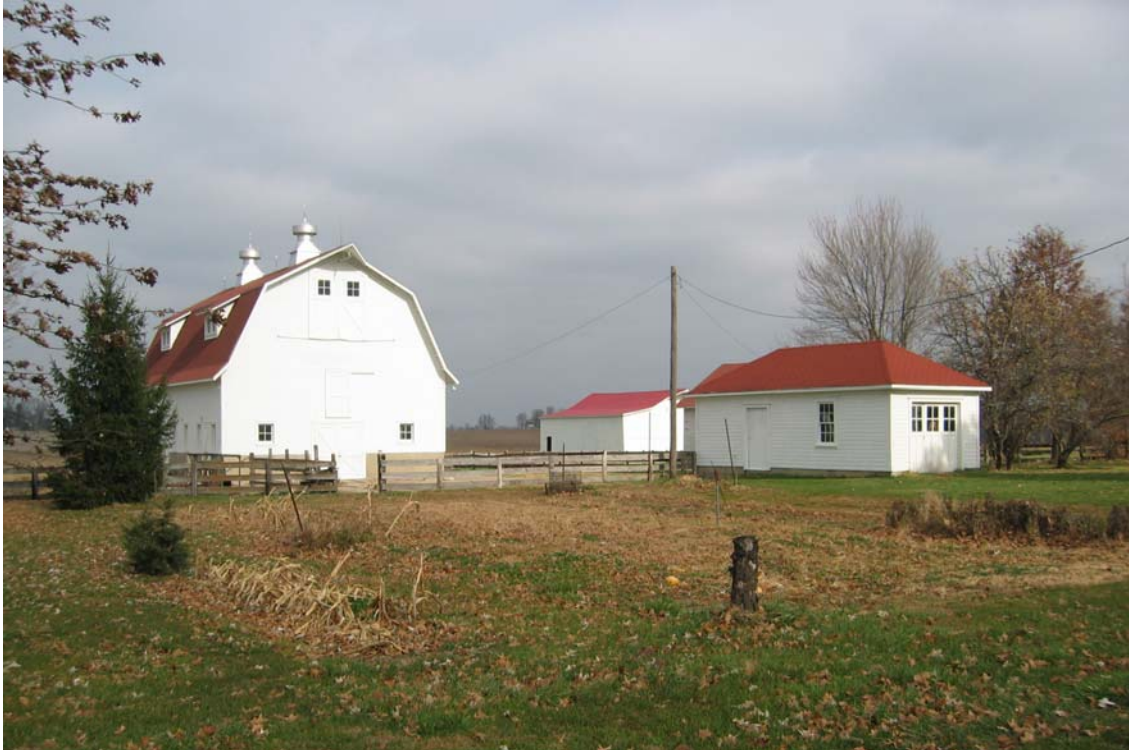
Figure 4. Outbuildings, Culbertson-Head Farmstead (November 2007). Jamesway barn is located on the left, nineteenth-century barn in the background. Adjacent to the Jamesway barn is the shop. View is northwest.
