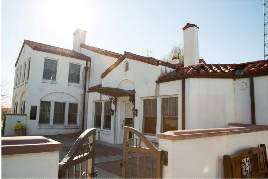
Figure 9: East elevation facing southwest. The patio in the foreground was added during the 2009 renovations.
