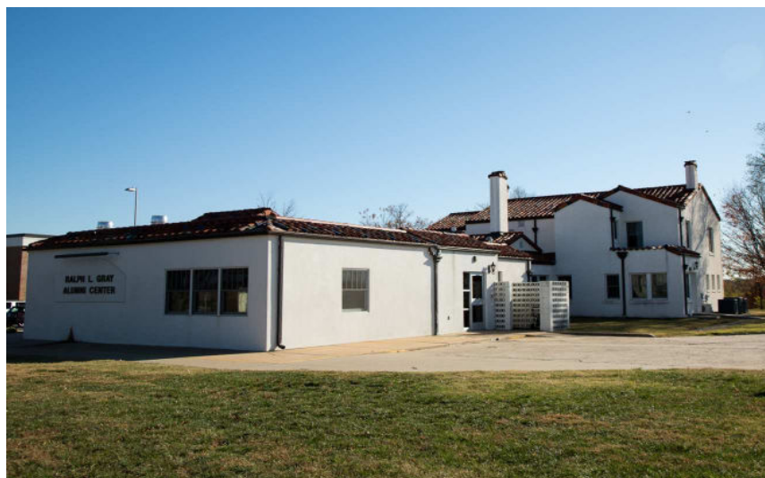
Figure 15: North and west elevations facing southeast.
