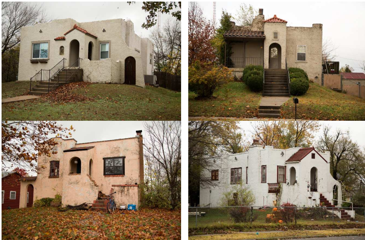
Figure 29: Photo Table of other Spanish Revival style homes in Joplin, Missouri. Clockwise from top left, 1326 Roosevelt Ave., 1417 Roosevelt Ave., 1505 Roosevelt Ave., and 1432 Roosevelt Ave. All homes are extant. All homes features arched, recessed entryways, tiled gable roofs over the porches, and flat roofs with parapets. The houses are in various states of disrepair, and none are as elaborate or ornate as the Buchanan residence. Additionally, none carry the low-pitch, tiled gable roof throughout the entire structure, like the Buchanan residence does. The homes are all located within the same two-block radius of Roosevelt Ave. Author photos: 2016
