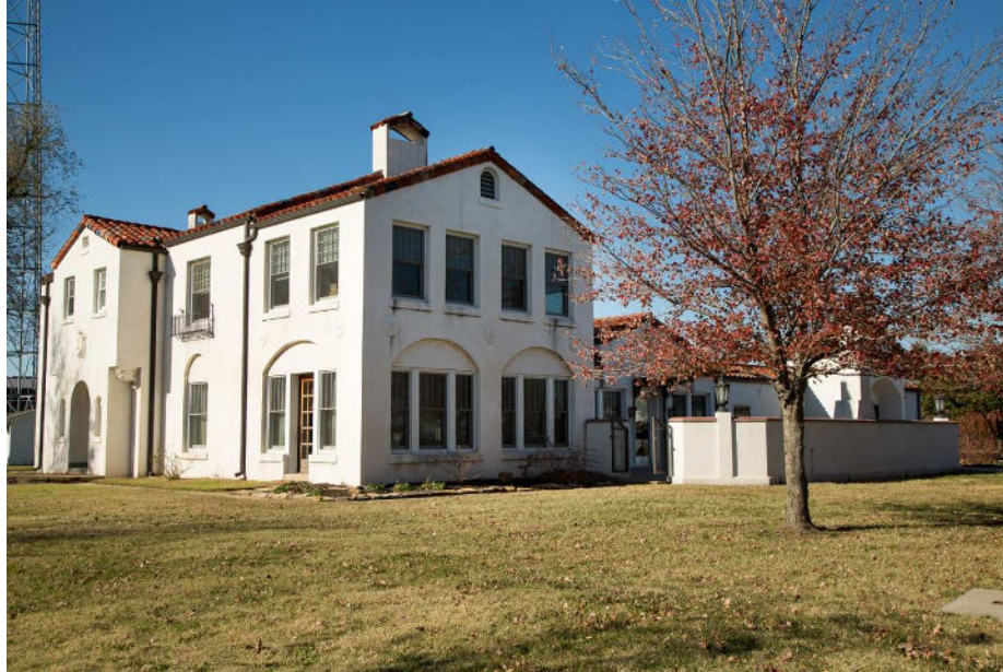
Figure 11: Southeast elevation facing northwest, approximately 50 feet back from the house.
