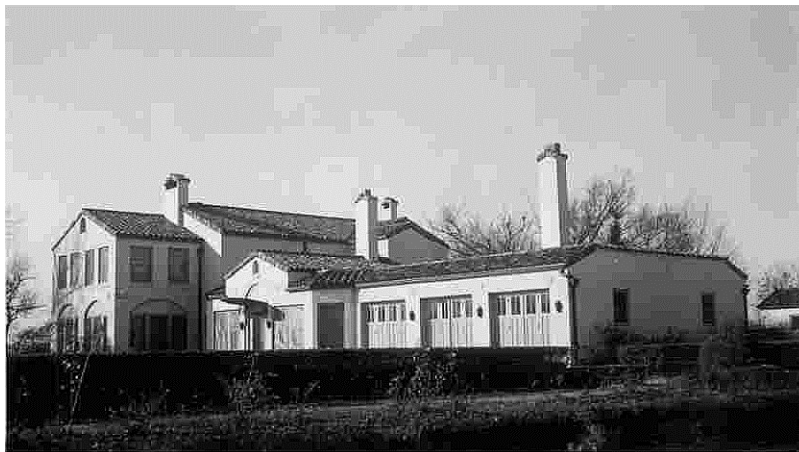
Figure 26: East elevation of house, facing southwest, c. 1940s. The original three-car garage can be seen on the right. Courtesy of MSSU Archives
