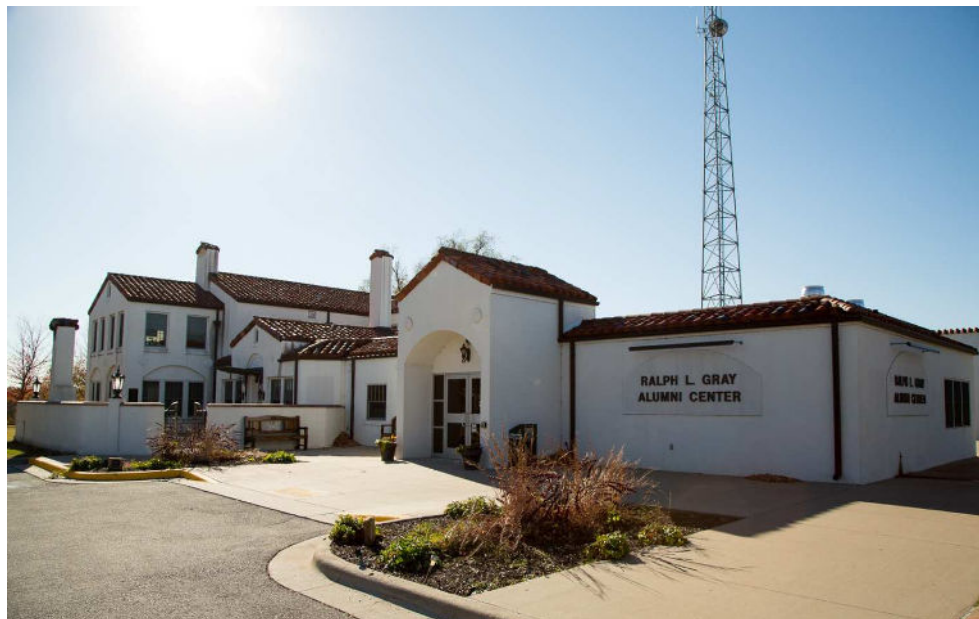
Figure 6: Northeast elevation facing southwest.
