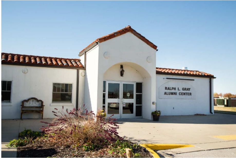
Figure 7: East elevation facing northwest. This photograph highlights most of the 2009 renovations, where this new space was created, taking the footprint of the former 3 car garage.
