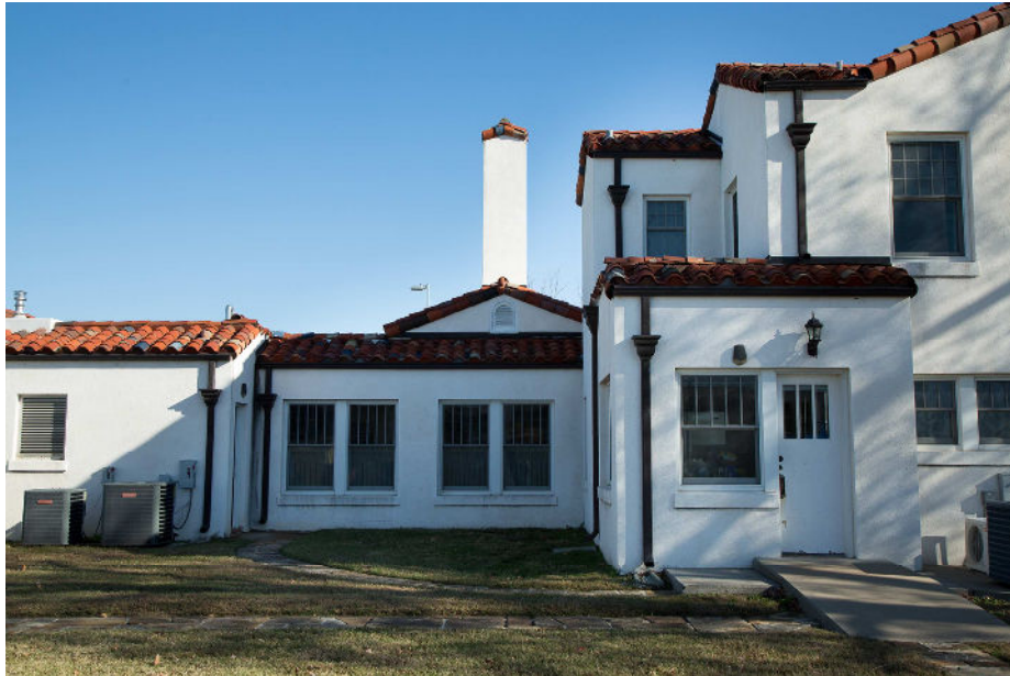
Figure 13: West elevation facing east.
