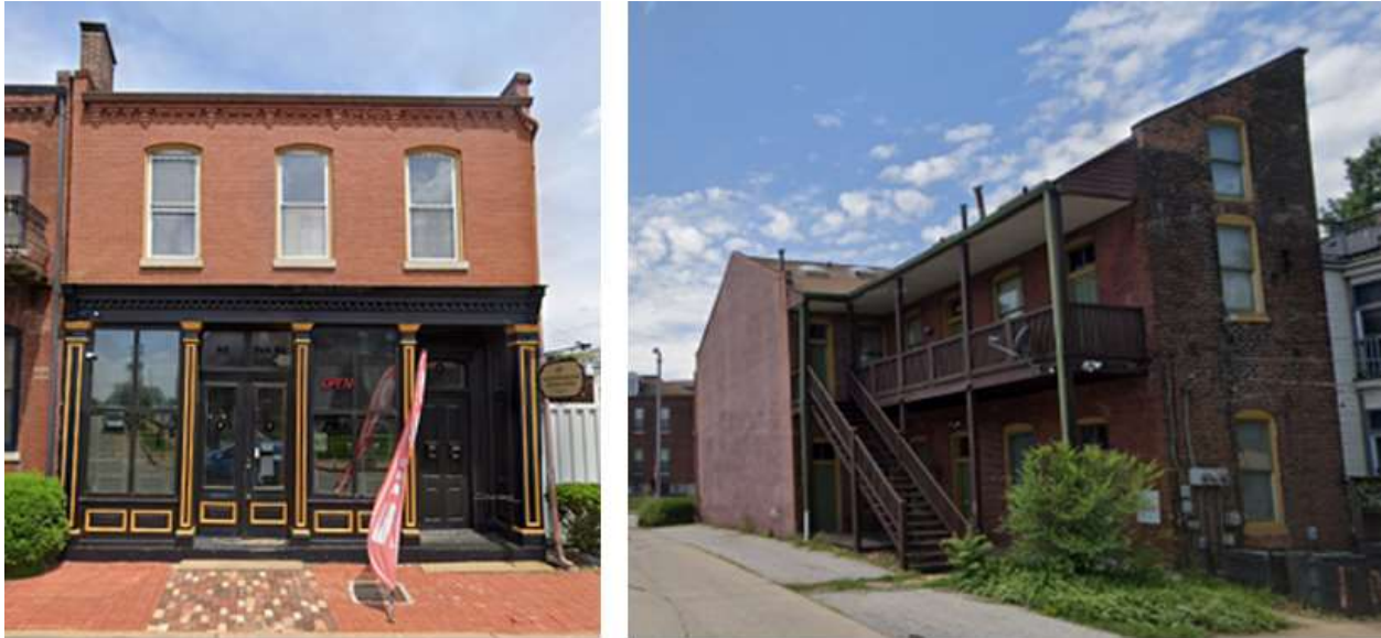
Above: A small number of extant flounders were built for mixed use with storefronts on the ground story and residential space above. This mixed-use building in the Soulard/Page District has a commercial storefront (left photo); at the rear is a flounder ell wing for residential use (right photo). It retains its historic gallery, which is accessed from the rear of the property, with a staircase to provide access to the upper level. Both photos from Google Earth.
