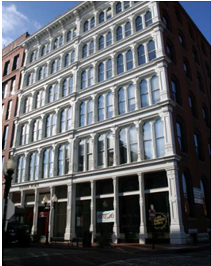
Above: Raeder Place was designed by German immigrant Frederick Raeder in 1874; it has a Victorian Italianate-style cast iron storefront. It originally housed the Christian Peper Tobacco Factory.
