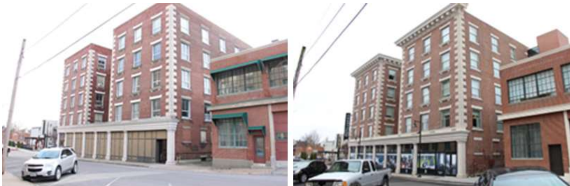
Left and Right: Before and After the 2016 rehabilitation of the H&H Building and the Rueseler Motor Company Building in Cape Girardeau. During rehabilitation a decorative parapet was returned to the H&H Building based on photographic evidence of its historic appearance.
