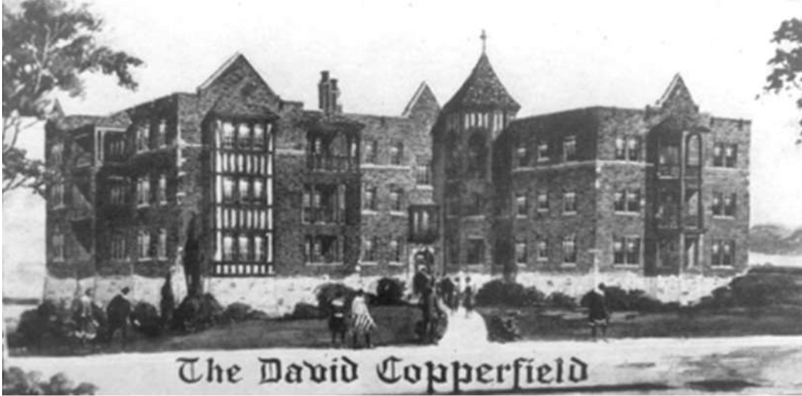
Image: Nelle E. Peters, David Copperfield Apartments, Kansas City, 1927, part of the “literary group” of apartment buildings adjacent to the Country Club Plaza
