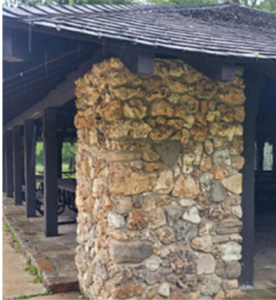
Exterior (left) and interior (right) of an Ozark rock masonry support wall of the Alley Pavilion at the NPS Alley Spring campground. The photo on the right shows typical "giraffe" construction with flat sandstone slabs.
