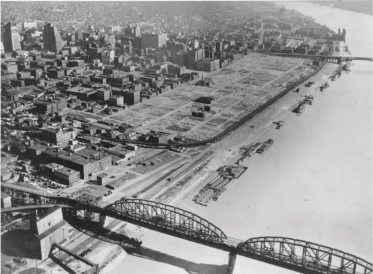
The St. Louis river front after demolition; Source: Jefferson National Expansion Memorial Archives, via Wikipedia
