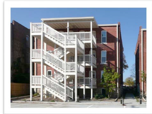
Top: Image of a deteriorated rear stair on a colonnade apartment building. Kansas City, MO, 2000. Below: Image of the new rear stair addition. The new stair was reconfigured to meet current building code requirements yet its design compatible with the historic structure. Kansas City, MO, 2000.
