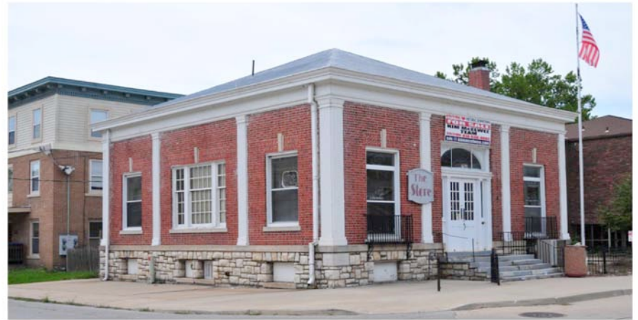
Example of a Classical Revival civic building, 339 East Broadway, 2014.
