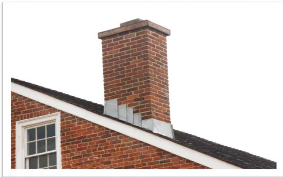
Example of roof flashing around a brick chimney, Howard County, Missouri, 2008.
