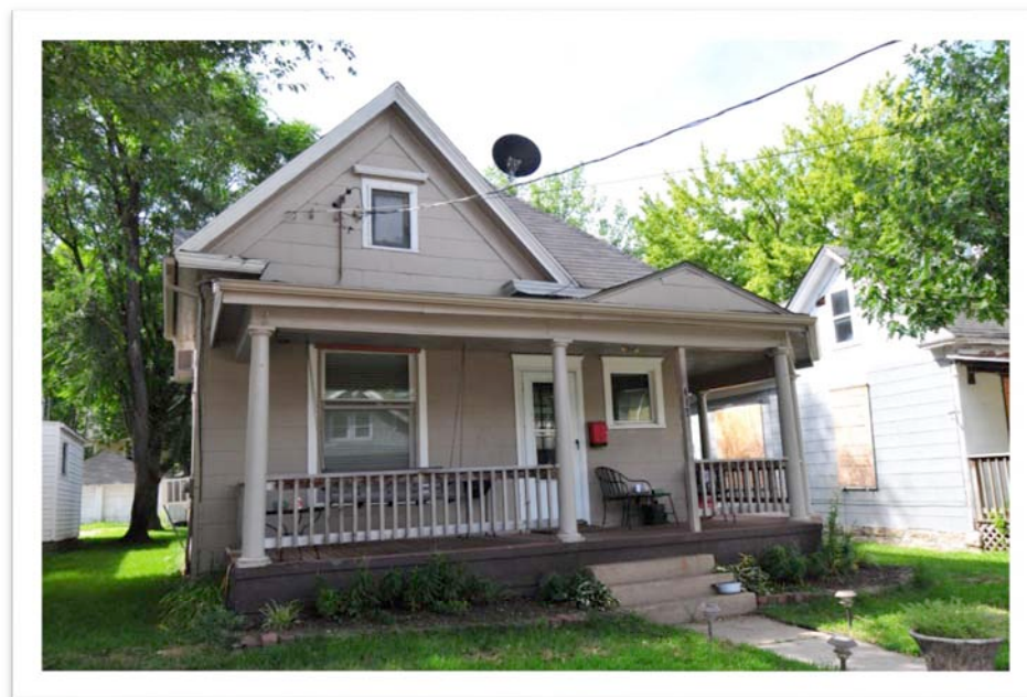
Example of Hipped Roof with Lower Cross Gable form, 417 Benton Avenue, 2014.
