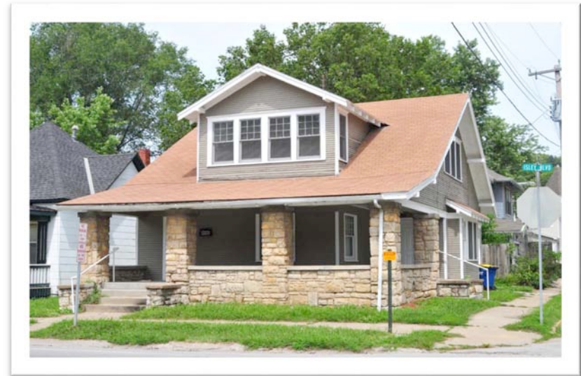
The masonry (stone) front porch of this Craftsman style home is an essential character defining feature, 432 Isley Boulevard, 2014.
