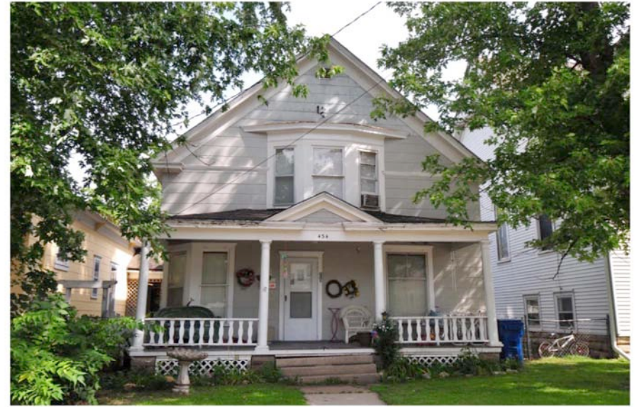
Left: 201 South Francis, 2014. Above: 434 Benton Avenue, 2014.
