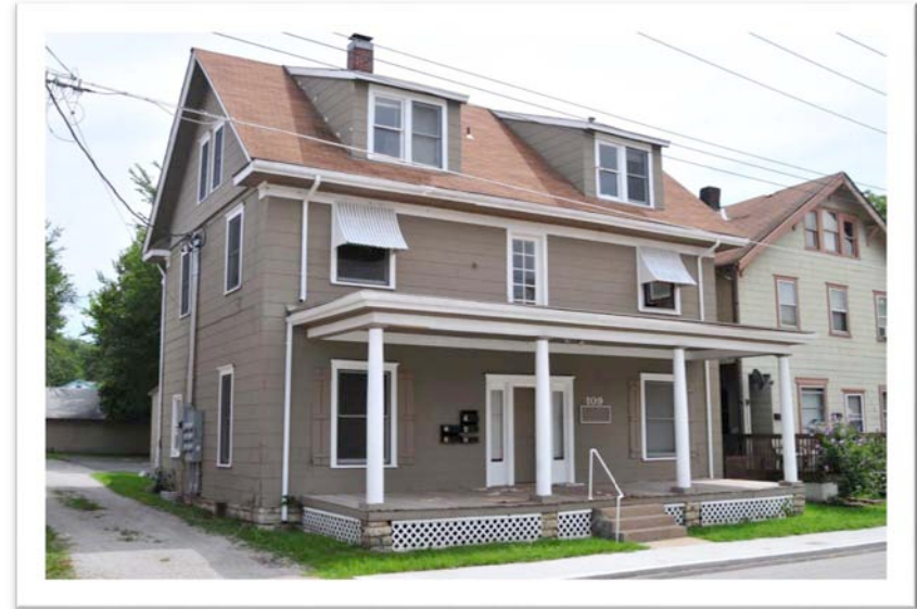
Example of painted metal awnings in good condition, 109 Saratoga, 2014.
