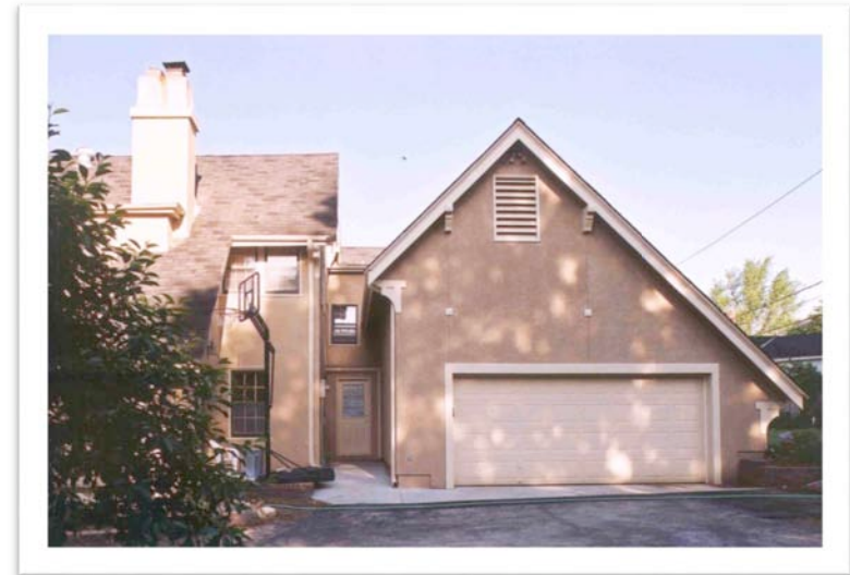
Example of traditional stucco installed on a new garage addition. Kansas City, MO, 2005.
