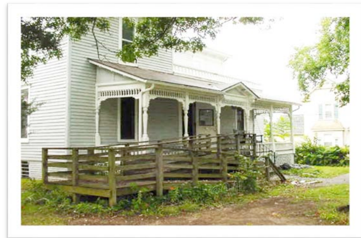
Top: Example of an inappropriate infill of a front porch. Bottom: Example of an inappropriate exterior ramp installation on the front of a historic house. The ramp design dominates the first impression of the house and does not resemble the house's style, nor is it painted to match.
