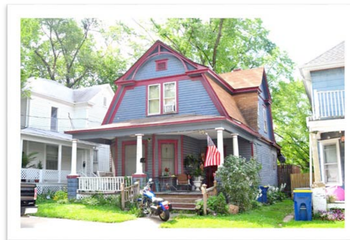
Top: 223 South Francis, Bottom: 515 Benton Avenue. Examples unique roof shapes that are character defining features that should be retained. Excelsior Springs, MO 2014.
