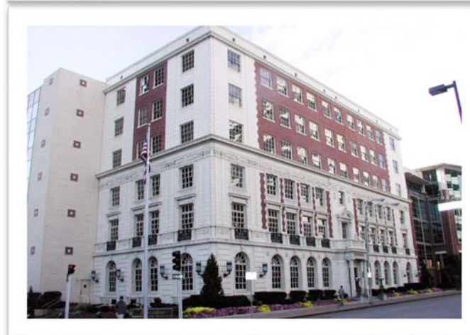
Top: Painted masonry building before paint removal. Kansas City, MO, 2004.
