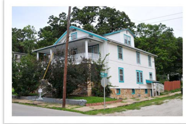
Below Left: Many of the houses in the district have exposed stone masonry foundations, 111 Temple, 2014.
