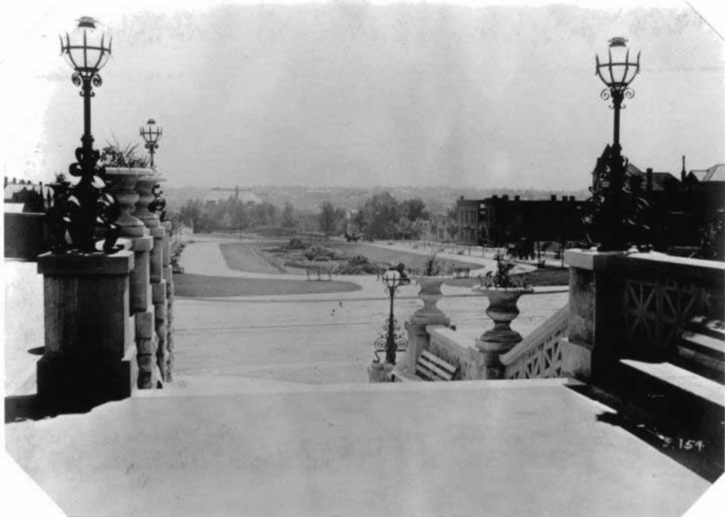
PS-6 Looking south from the Terrace
