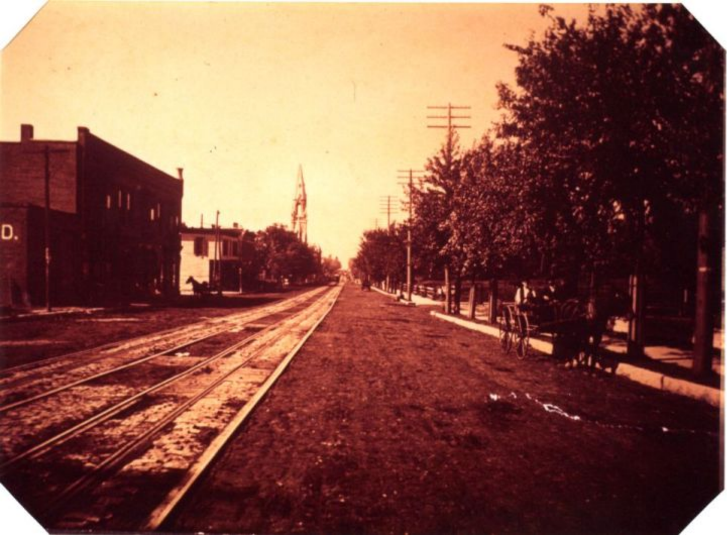
I-1 Independence Blvd. @ Montgal Av., West 1894
