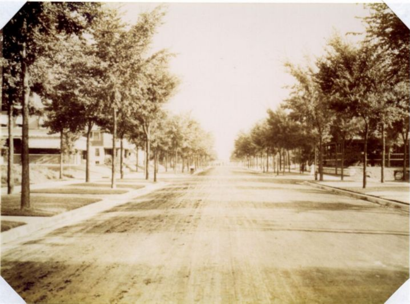
I-5 Gladstone Blvd., North of Thompson Av. 1909
