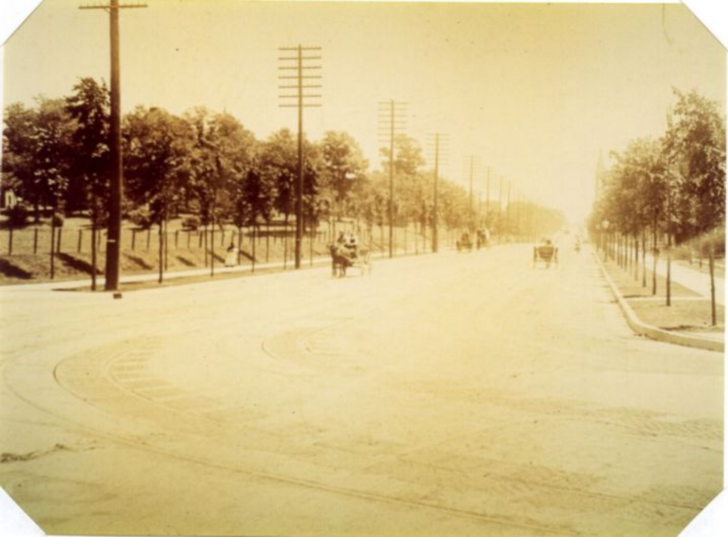
I-3 Gladstone Blvd. @ Anderson Av. 1899
