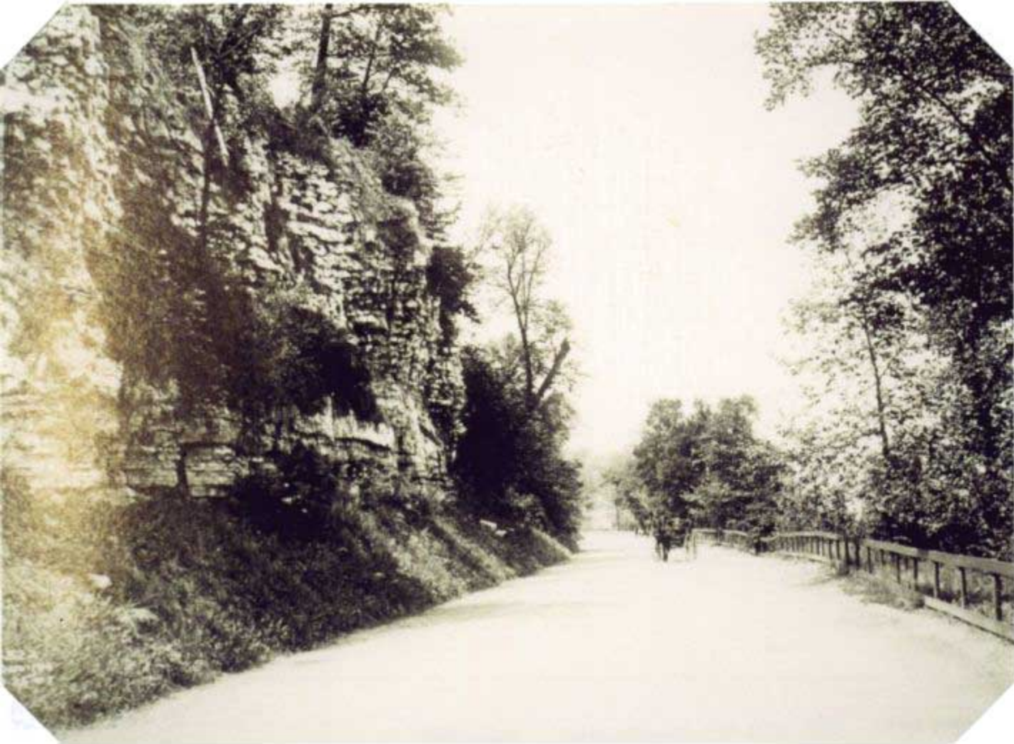
K-20 Cliff Drive at Scarritt Point 1907
