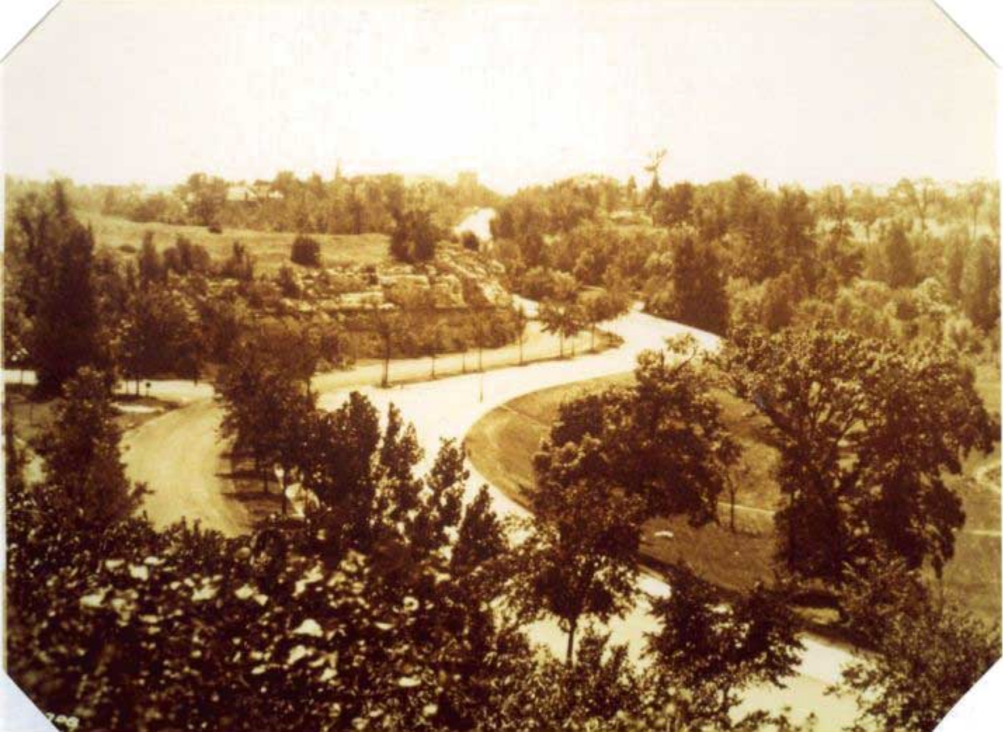
PV-4 28th & Broadway, looking south 1914
