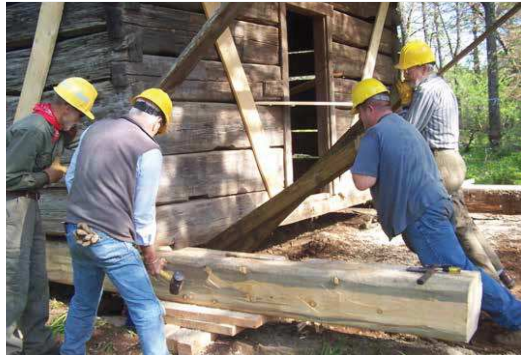
ABOVE: Cabin at Falling Springs, Mark Twain National Forest
